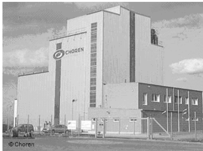
Fig. 16: Industrial syngas production plant, Choren GmbH, 2003
