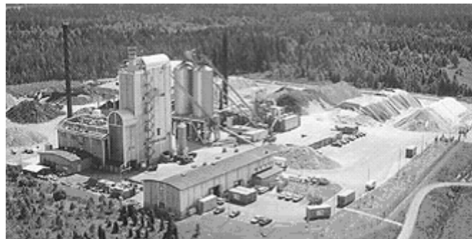
Figure 18 Värnamo IGCC plant
