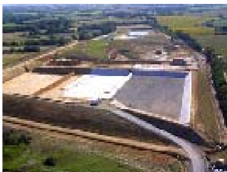
Figure 4 : Photo of the bioreactor cell before its filling
