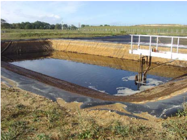
Figure 11: Photo of the lagoon reserved for the bioreactor
