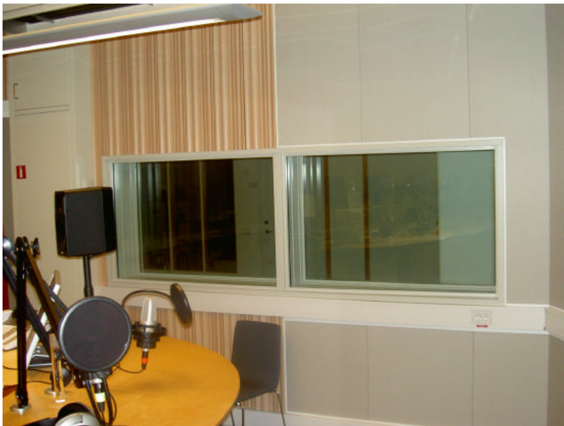
Figure 6.11. The non-preferred room, control room aspect, side view showing Svanå miljöteknik AD10 diffuser panel to the left and Ecophon Wall panel to the right. The windows are splayed horizontally.
