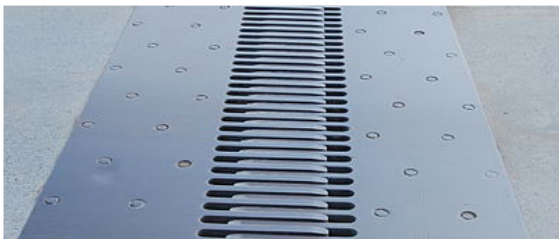
Figur 13. Expansion joint in a steel plate girder bridge (Wade, 2009). CC BY-SA.
