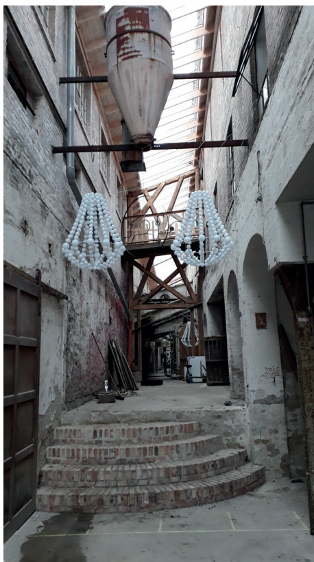
north-side light-corridor renovated with recycled bricks from the factory and up-cycled metal for bridges
