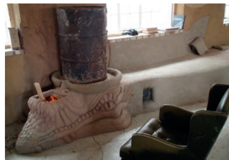
rocket stove built with recycled bricks from the factory and using clay render
