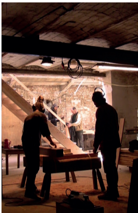
sharing carpentry knowledge while learning to build a wooden staircase
