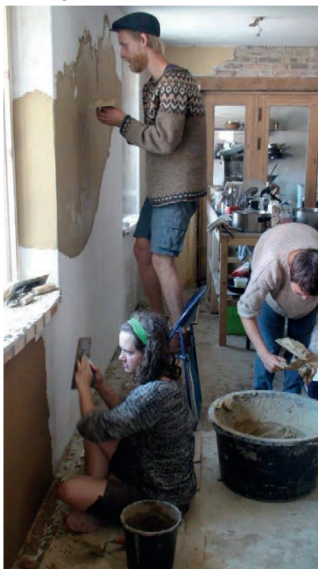
learning together clay and lime rendering technique with natural pigments
