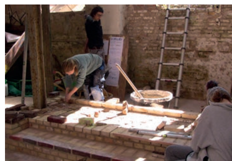
sharing bricklaying knowledge while learning to build a staircase with recycled bricks from the factory and using clay mortar
