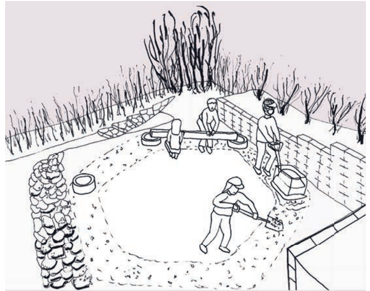
Figure 45. Preparing the ground for building the foundation
