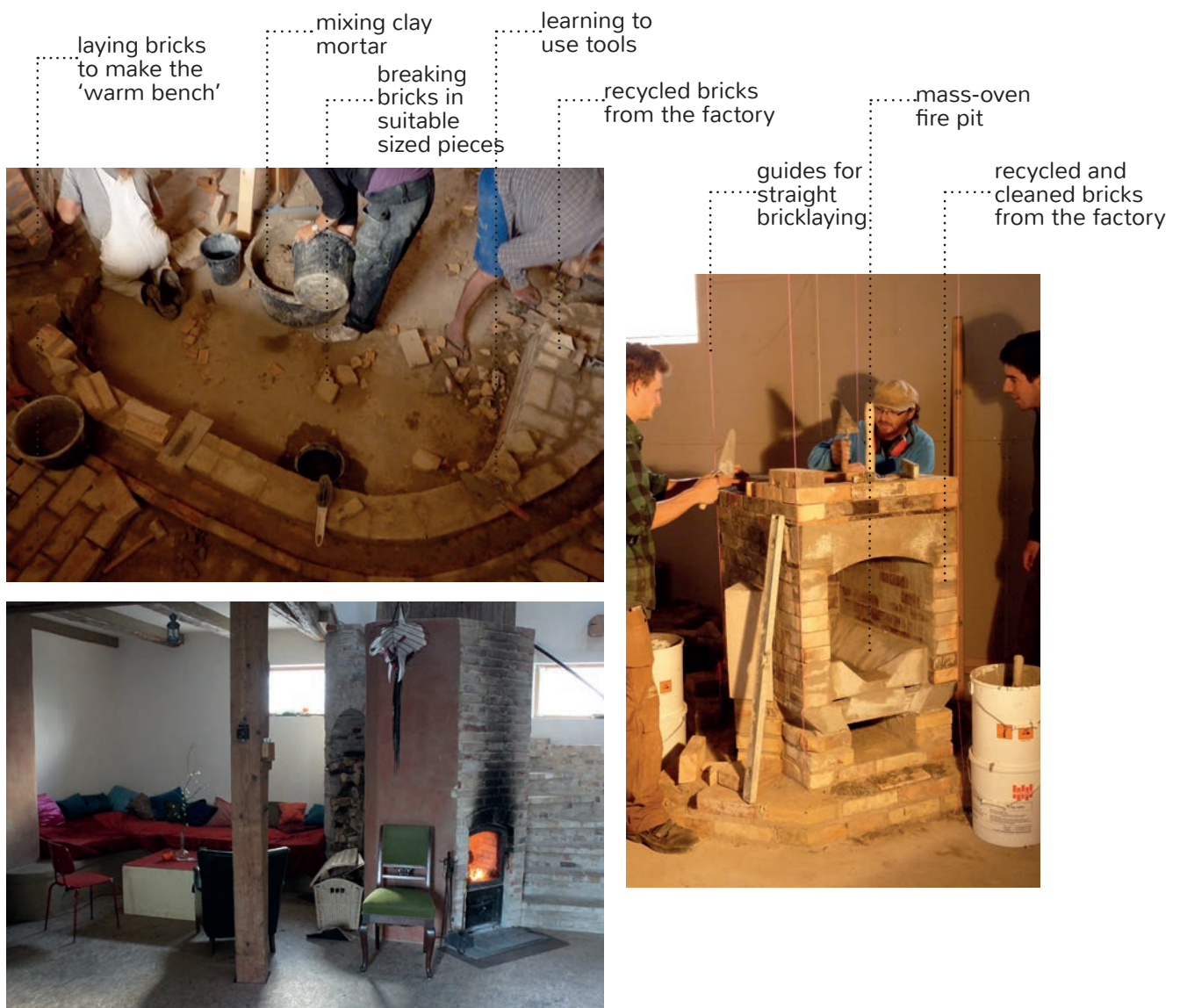
Figure 21. Photos of Makvärket 'building a mass-oven'
