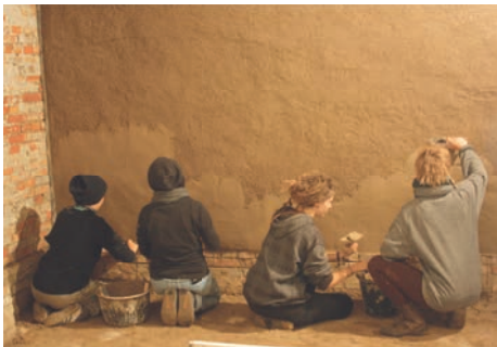
2012 applying clay-render to walls
