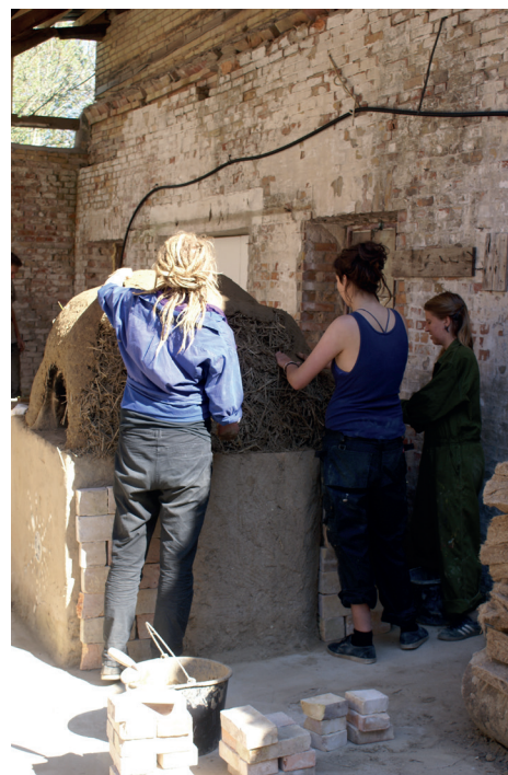
learning together the cob technique while building a pizza oven
