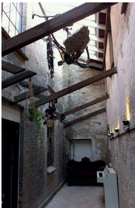
south-side light-corridor renovated with recycled bricks from the factory
