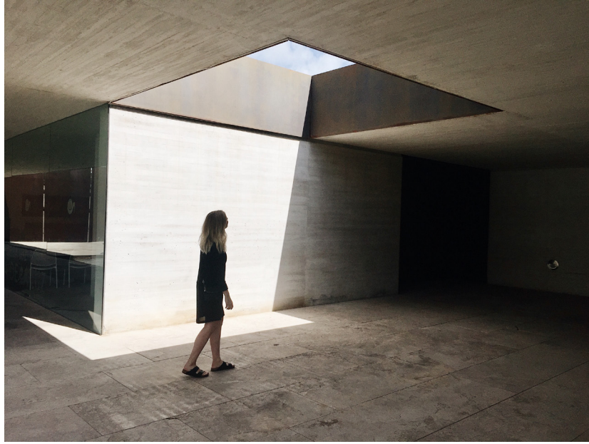
Figure 24. Solar heat load: Nieto Sobejano Arquitectos, Castillo De La Luz Museum, Las Palmas de Gran Canaria, Spain, 2013. A concrete slab protecting the fully glazed entrance hall from the sun, with an opening to let light in. Author's own image.
