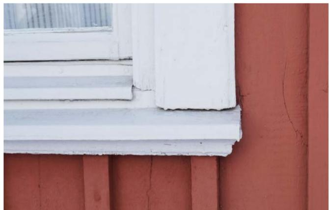
Figure 44. The sill of a window.
