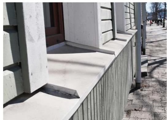
Figure 71. Sill of a window that rests on a level-ribbon.
