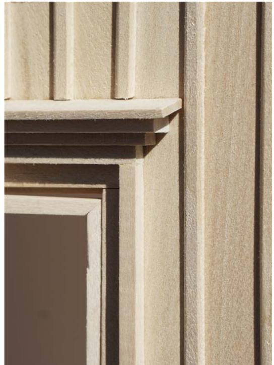
*Figure 124.* Head casing of window at entrance floor. Different depths of the casing. Original scale 1:10.
