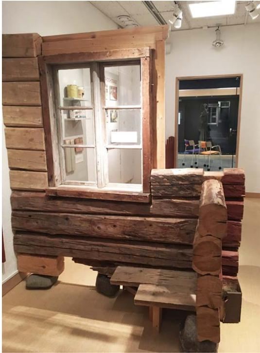
*Figure 15.* A timber wall without panelling.
