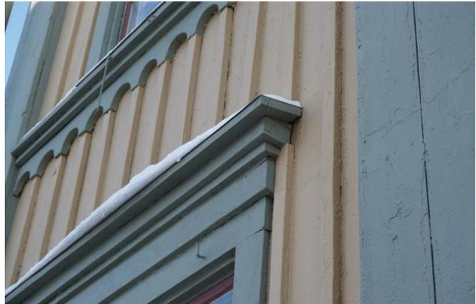
Figure 53. The headcasing of the window on the first floor.
