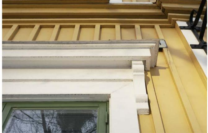
Figure 49. Head casing of a window.
