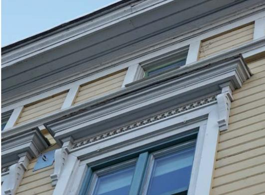
Figure 59. Profiled head casing of a window.
