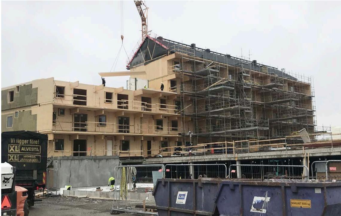
Figure 2. Construction of a multiresidential building in cross laminated timber, Växjö.
