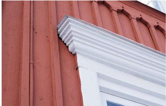
Figure 43. The head casing of a window.
