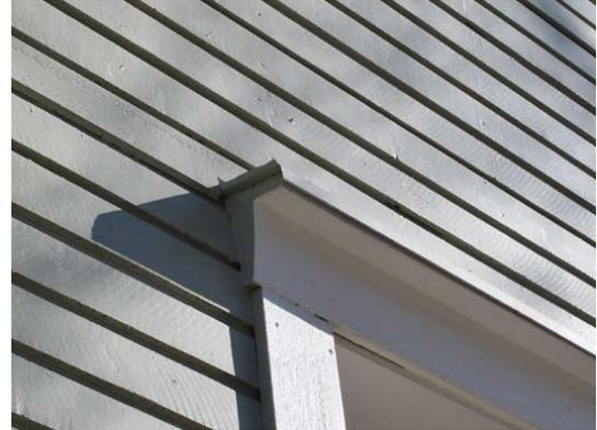
Figure 70. Head casing of a window.
