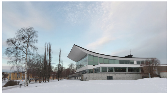
Winter view of the eastern facade and southern facade.
