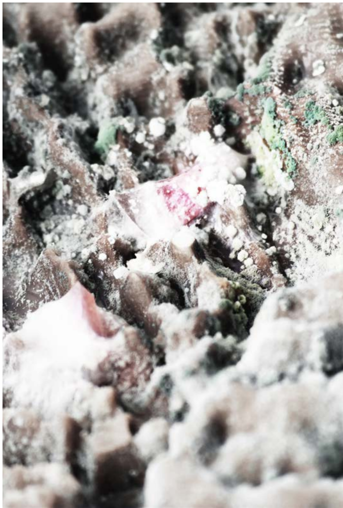
Geometry overgrown by the green mould.
