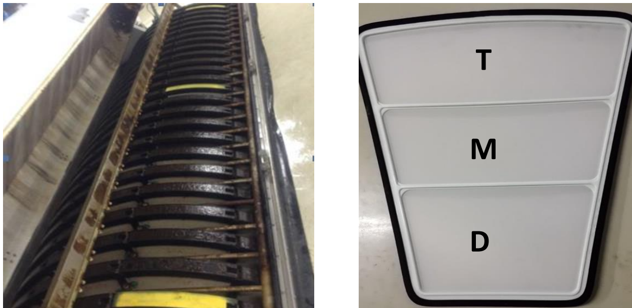
Figure 7 Discfilter at Trollhättan treatment plant and a discpanel showing different regions
