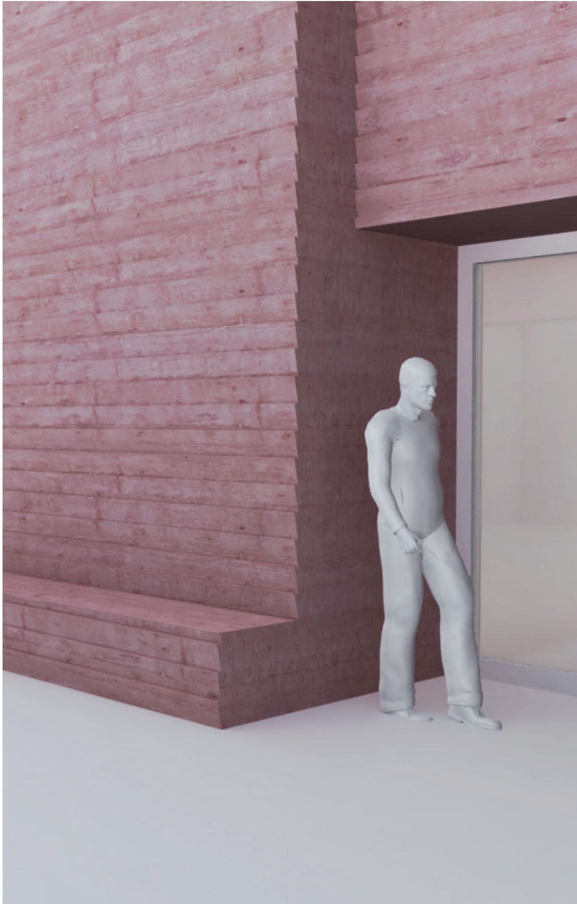
Fig. 53. Concrete cast in clapboard formwork. (Author's own copyright.)
