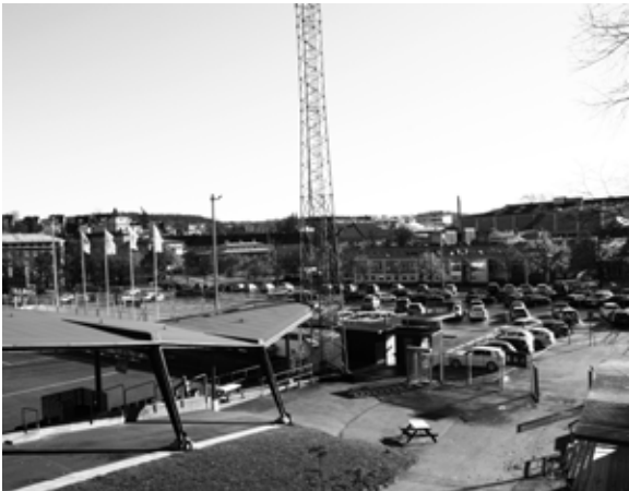
The current central bath is also made of bricks.
