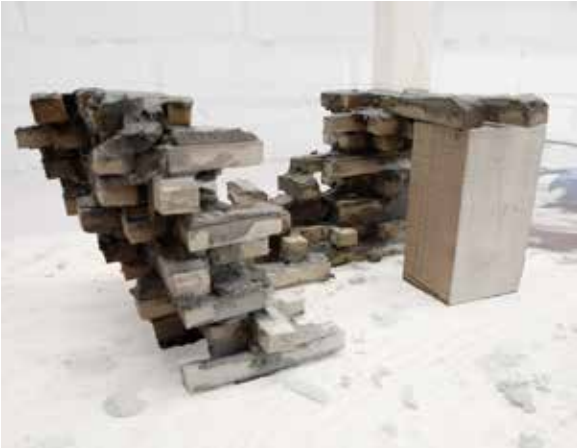
5. A support was placed below cantilevered parts to resist tension during construction
