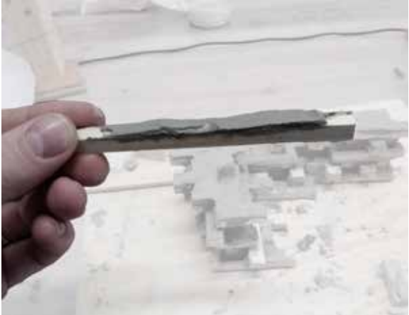
2. Depending on the situation, mortar was applied either on the brick or on the course below.
