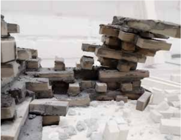
5. When structure started to cantilever it could no longer withstand the tension
