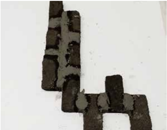
1. first course. Bricks gets soaked and soft.
