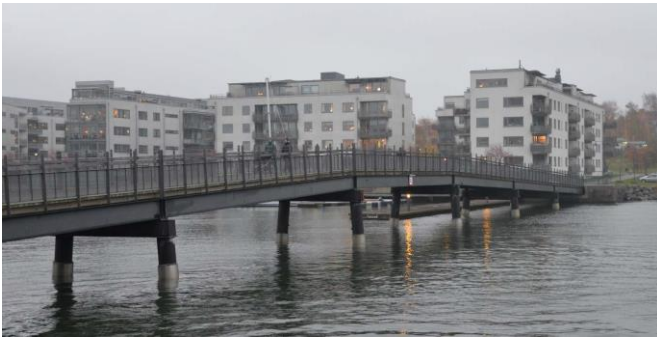
Fig. 1. Photograph of the pedestrian bridge analyzed in the project.
