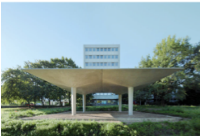
Figure 4-1. Pavilion at Aachen University made of a roof structure of TRC. (Photo: Bauko 2, RWTH Aachen University) (Scholzen et al., 2015).
