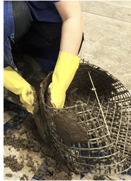
Figure 8-18. Apply concrete on the reinforcement (Photo: Johanna Riad)
