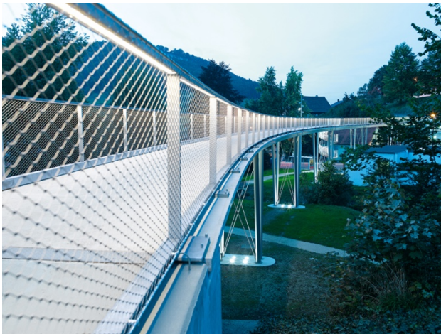
Figure 4-2. A 100-meter-long pedestrian bridge in TRC, is today the longest bridge built in TRC. (Photo: InnovationsinTextiles 2011)
