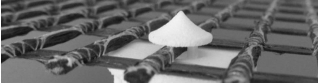
Figure 3-4. A spacer can be added at the reinforcement to guarantee right place and distance. This one is from DistTEX (Photo: DistTEX)
