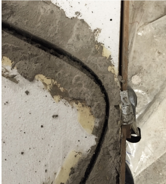
Figure 9-10. Deformation of formwork causing thinner parts. (Photo: Ellen Simonsson)
