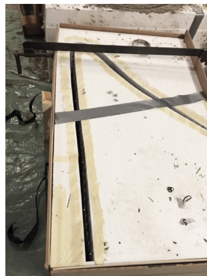
Figure 9-8. Clamps to stabilize the formwork. (Photo: Ellen Simonsson)
