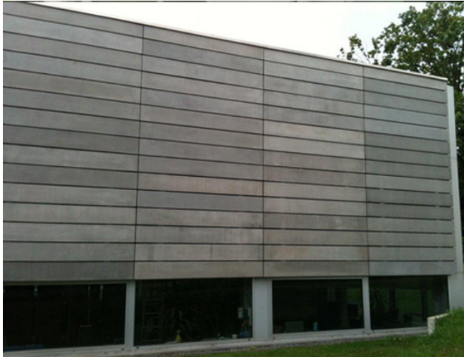
Figure 4-3. Façade elements of TRC.
