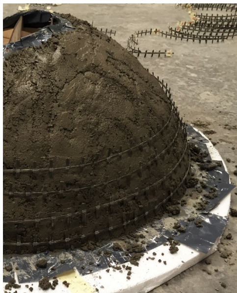
Figure 8-11. Horizontal reinforcement placed over one layer of concrete. (Photo: Ellen Simonsson)
