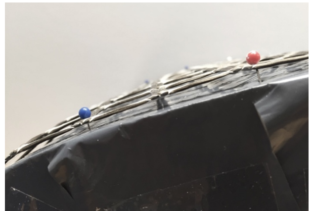
Figure 8-2. Below: With nails the reinforcement was placed in right distance from foam formwork. (Photo: Ellen Simonsson).
