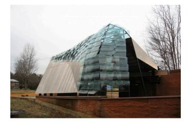
Fig. 23. The Manson Bend Glass Chapel by Rural studio with layered glass facade made of thrown away car windscreens. The shape of Rural Studios project usually grow from experiments with materials at hand.
