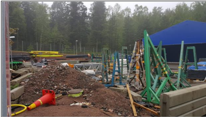
Figure 5.11 Earth that is disposed on the construction site
