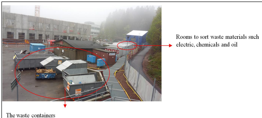
Figure 5.3 The location of waste containers
