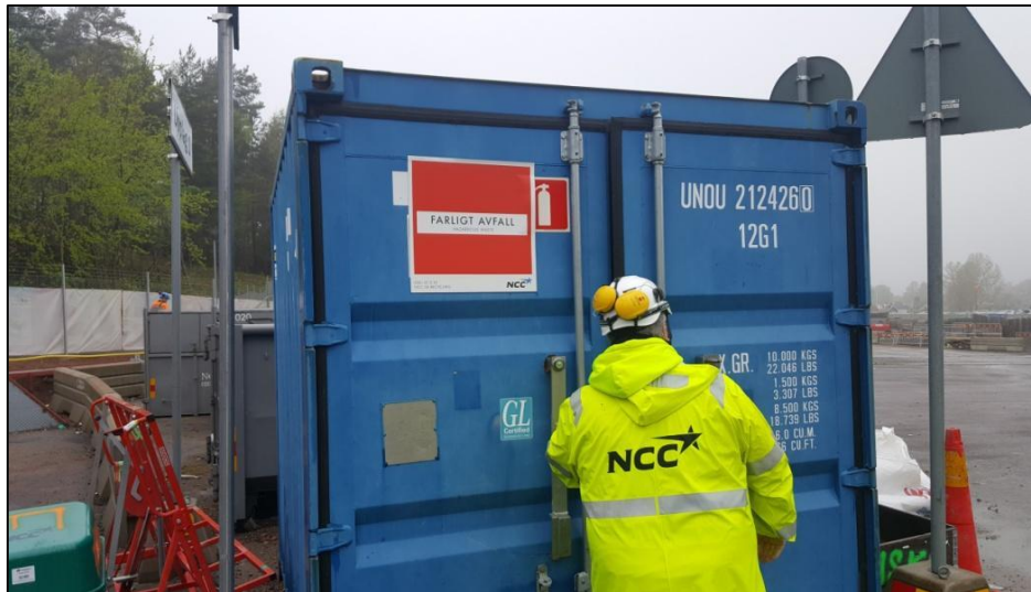
Figure 5.5 Waste Container is signed with red colour for hazardous wastes
