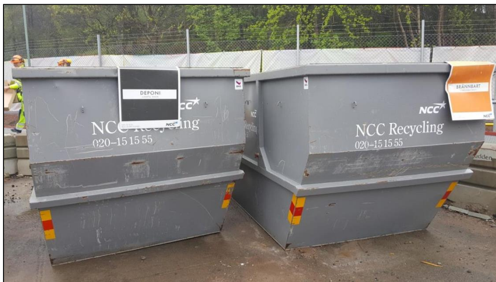
Figure 5.4 containers with orange and red colour tag for combustible and landfill wastes
