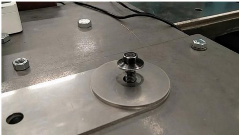
**Figure 4.7:** A large washer between the bolt and the component.
