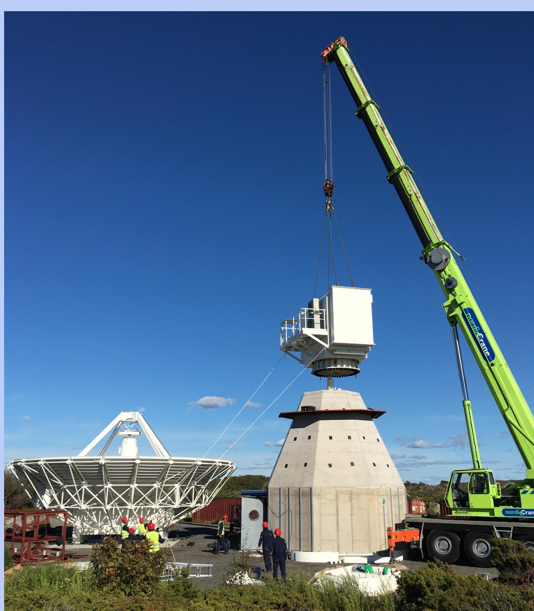
Lifting the azimuth cabin of the southern telescope.
