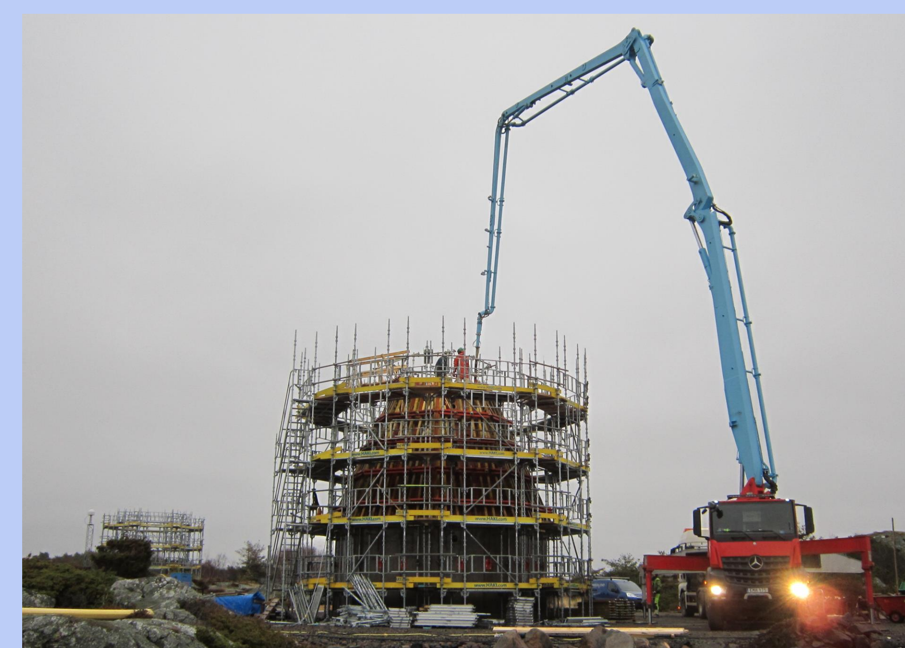
The concrete foundation of the southern telescope.
