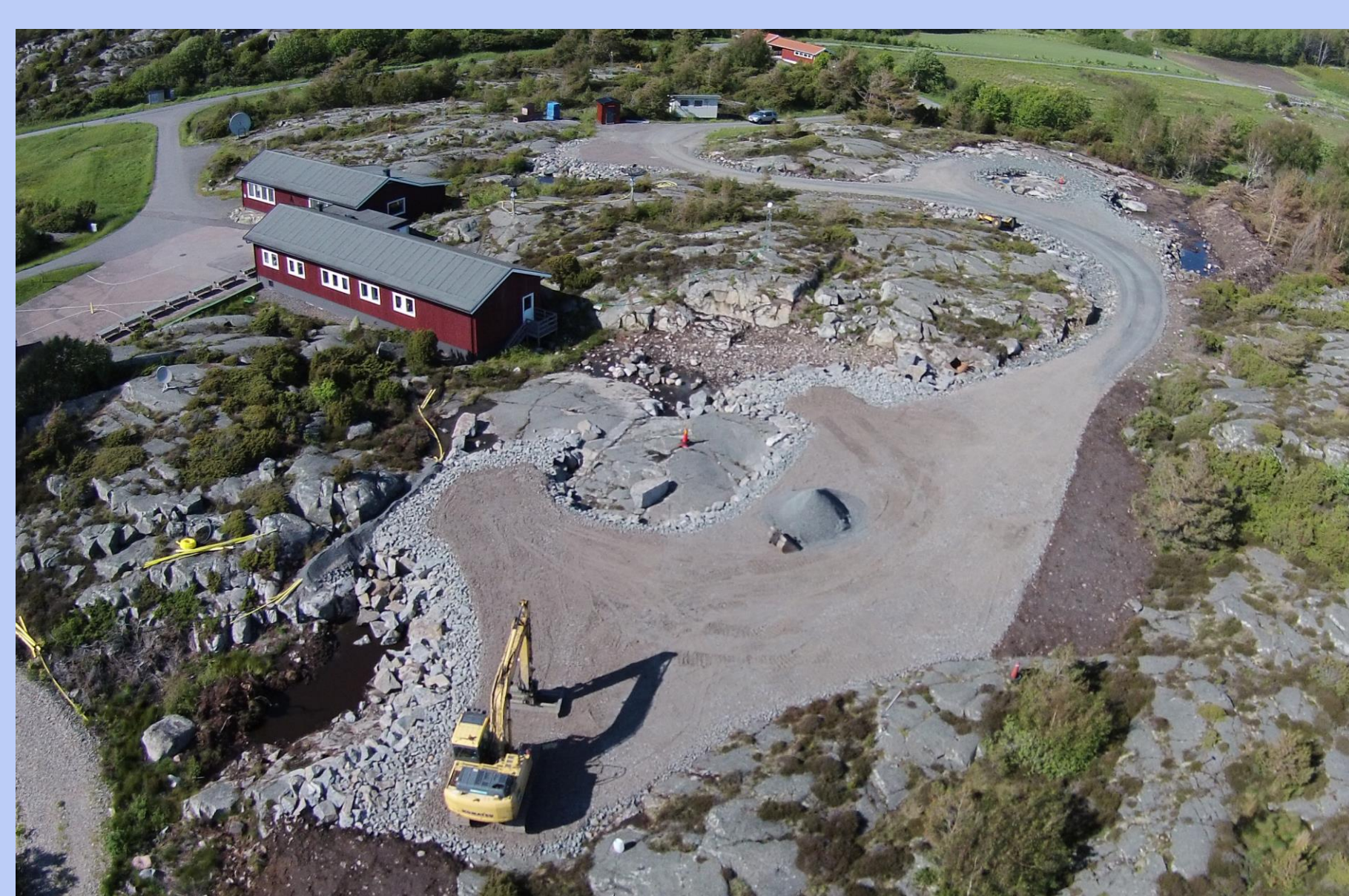
Ground preparations almost ready.
