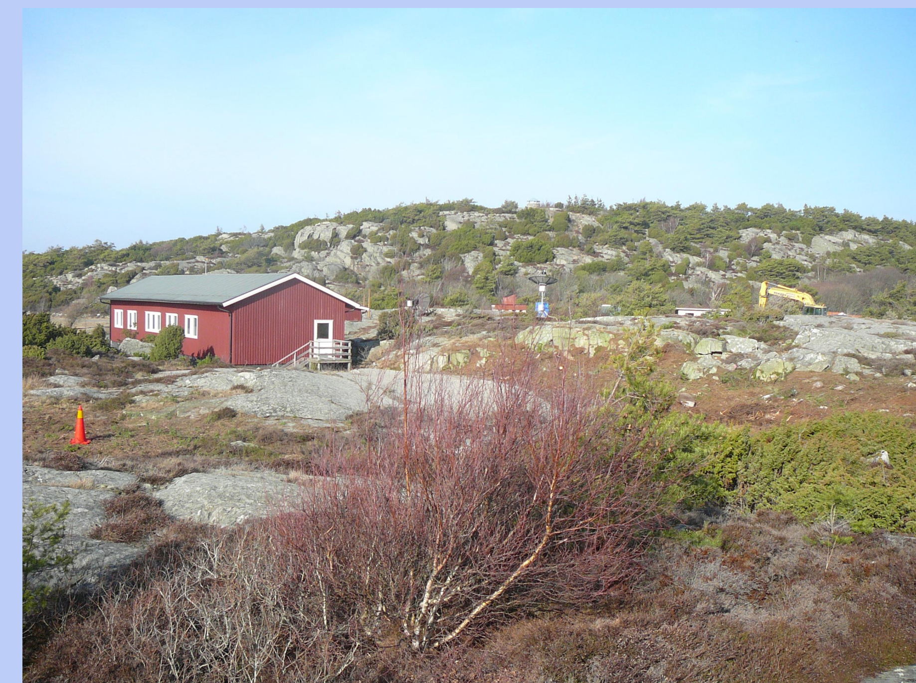
Preparing the grounds in February 2014.
