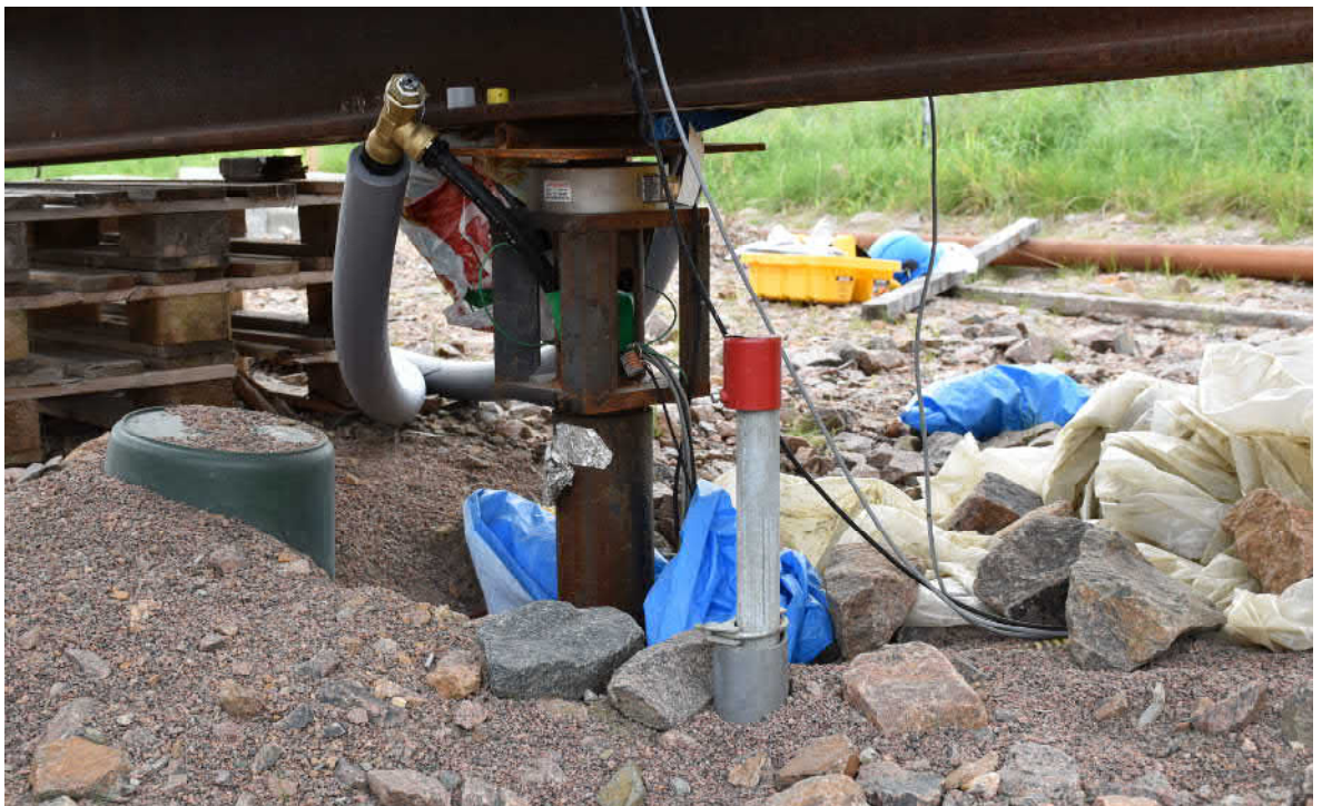
Figure 2. Pile head of the steel thermal pile at Utby with U-tube heat exchanger, fibre optics for distributed temperature sensing, and cables, before final insulation. The pipe with a red cap is the head of a bellow hose used for settlement measurement. Below the bucket to the left is a station of 4 pore pressure and temperature sensors (BAT). A pressure cell for measuring data on static load is placed between the pile head and the steel beam on top.
