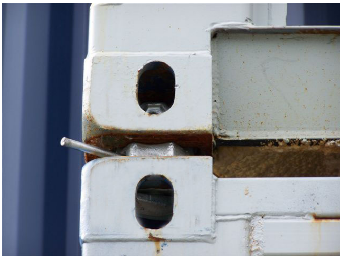
Figure 2 manually locked twist lock between containers (Göteborgs Hamn Bildbank, 2016)
