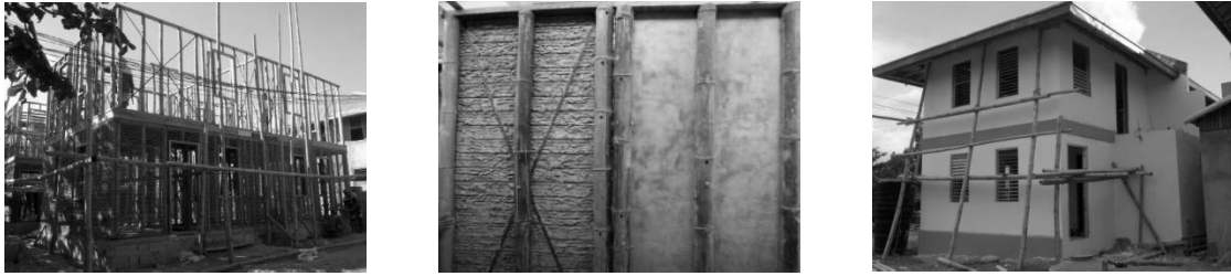
Picture 6: Modern bamboo-based housing built in Iloilo, Region IV in 2015 by [19], [27]
