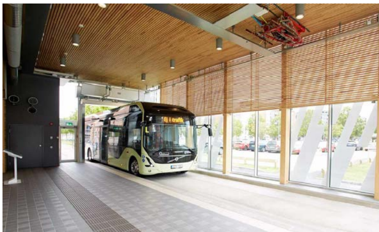
Fig. 1. The electric bus drives through the entrance to the indoor bus stop at Lindholmen.
