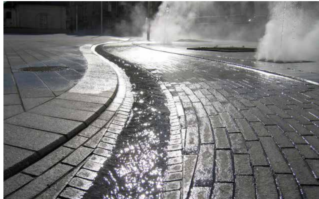
Open storm water channel highlighting water flow in Le Creusot, France (Llorca, n.d.)
