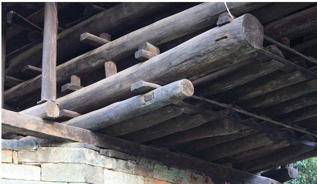
Figure 2.19 Chengyang Bridge stacked beam base, Sanjiang, China [10]
