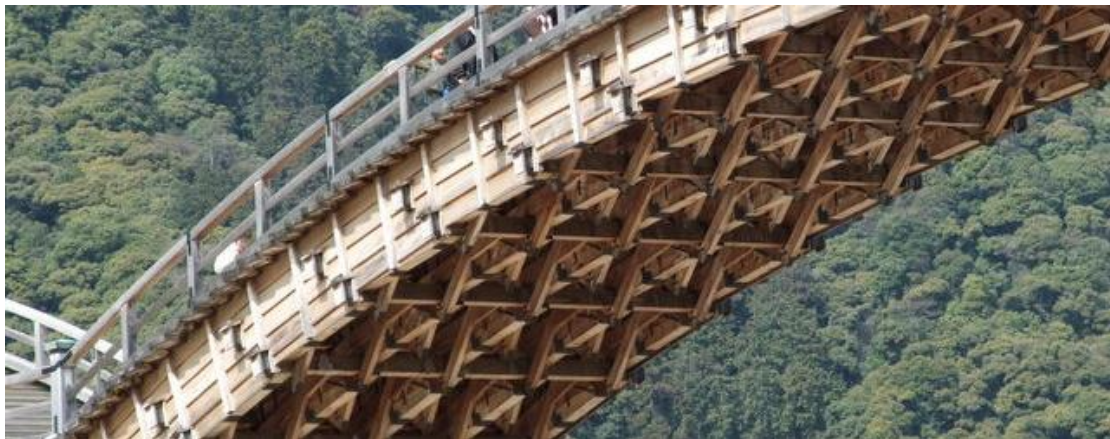
Figure 3.8 Structure of Kintai Bridge, Iwakuni, Japan [22]
