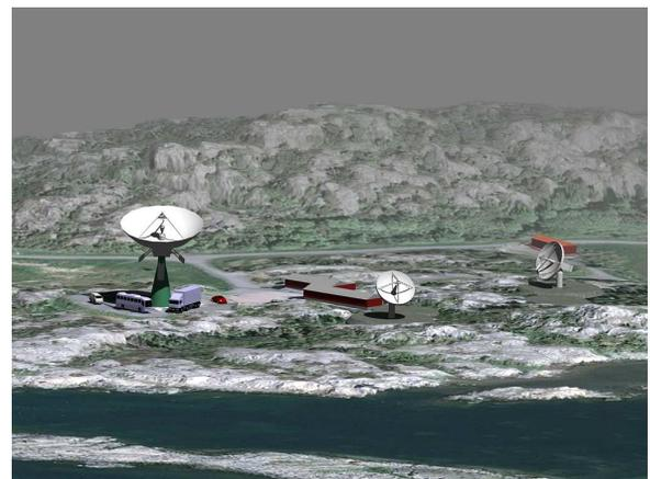
**Fig. 1** An artist's impression of the planned Onsala Twin Telescope (the two smaller antennas on the right side) together with the existing 25-m antenna (left). This is the new updated proposal of December 2013.
