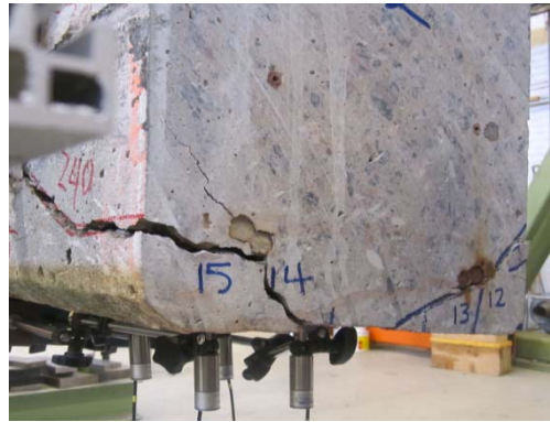
Medium damaged M2
