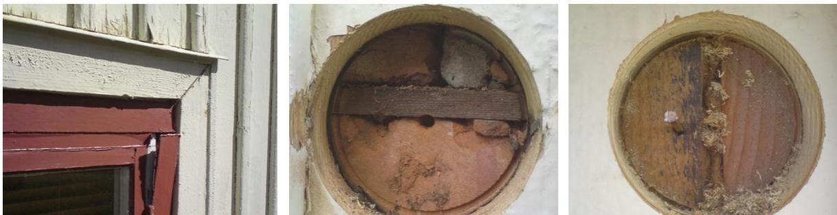
*Figure 4.2. At a visit to the buildings, holes were drilled through the wooden cover board to investigate the condition of the materials behind. The worst places were around windows (left) and in the wooden laths found in the grout between the bricks (middle). The wooden planks had flax between the planks (right) to increase the air tightness of the wall.*
