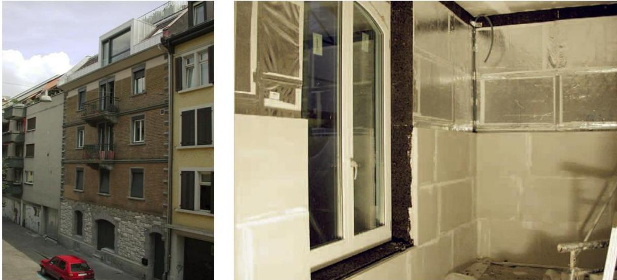
Figure 2.11. Interior insulation of a brick masonry wall in Zurich, Switzerland using 30 mm VIP covered by 60 mm plaster boards (Photo: Viridén + Partner AG).
