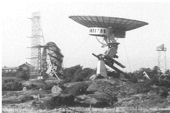
**Fig. 2** Two of the parabolic antennas at Onsala in the 1960'ies. Right: The 12 m diameter telescope ("nr. 1") that was destroyed in a storm in 1969. Left: A 9 m diameter Würzburg antenna ("nr. 2"). The antennas formed a west-east baseline ("nr. 2" to "nr. 1"). The photo is taken from Rydbeck (1991).
