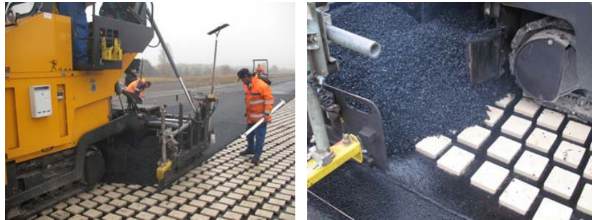
FIGURE 8. Pictures of the laying process.
