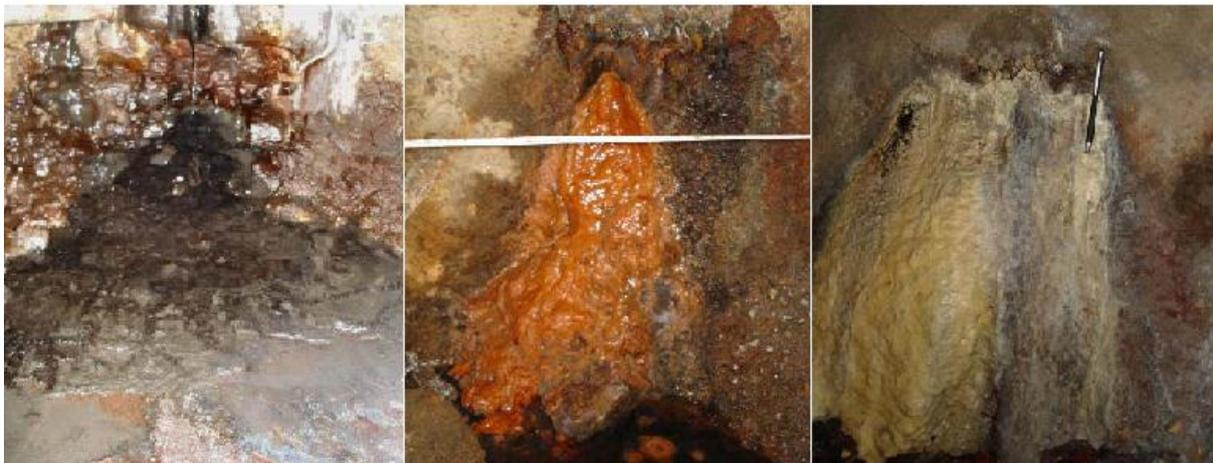
*Picture 1: Left picture shows precipitates of manganese, middle picture displays precipitates of iron and the right picture shows calcite precipitates contaminated by iron (Ekliden, 2008).*
