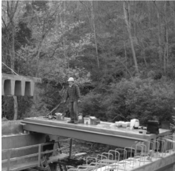
Figure 4.26 Example of FRP bridge elements with T-section, SuperFiberSPAN™, from Composite Advantage (2011)
