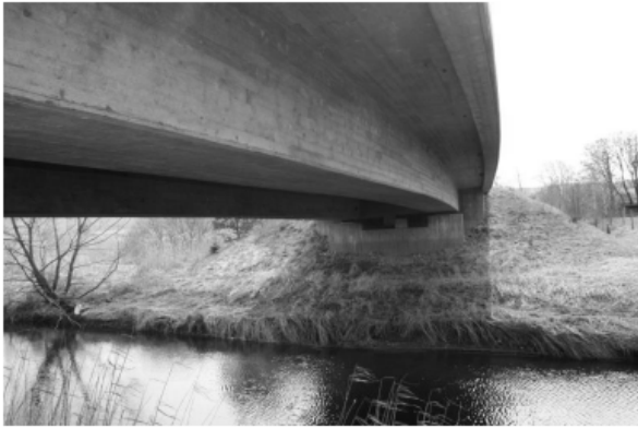
Figure 4.8 Beam bridge, box cross-section, from Ehlorsson, V.; Palmqvist, V. (2010)
