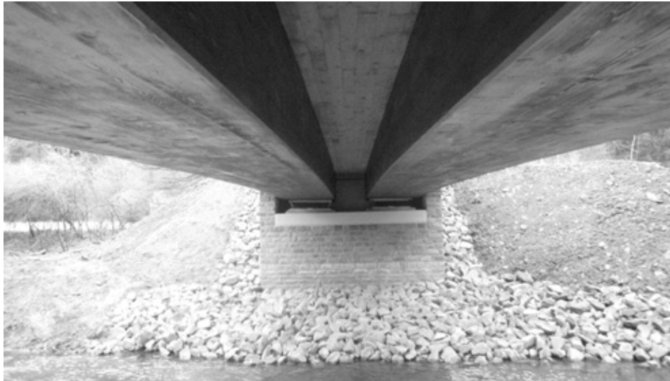
Figure 4.27 Example of composite bridge from Germany, property of Miebach Ingenieurburo (2011).
