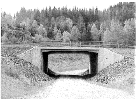
Figure 4.1 Typical slab-frame concrete bridge, from Vägverket (2006)
