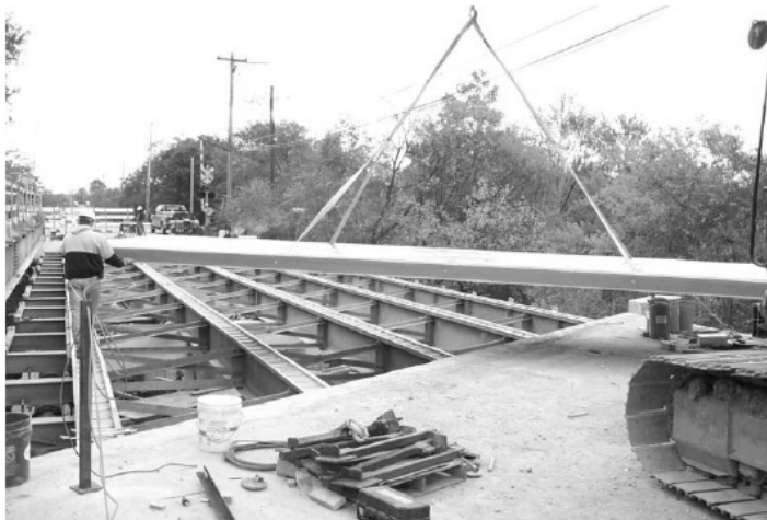
Figure 4.25 Example of FRP deck panels (FiberSPAN™) panel placed on steel grid, from Composite Advantage (2011)
