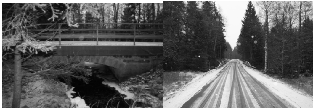
Figure 6.1 The Backaå bridge (Ramböll)
