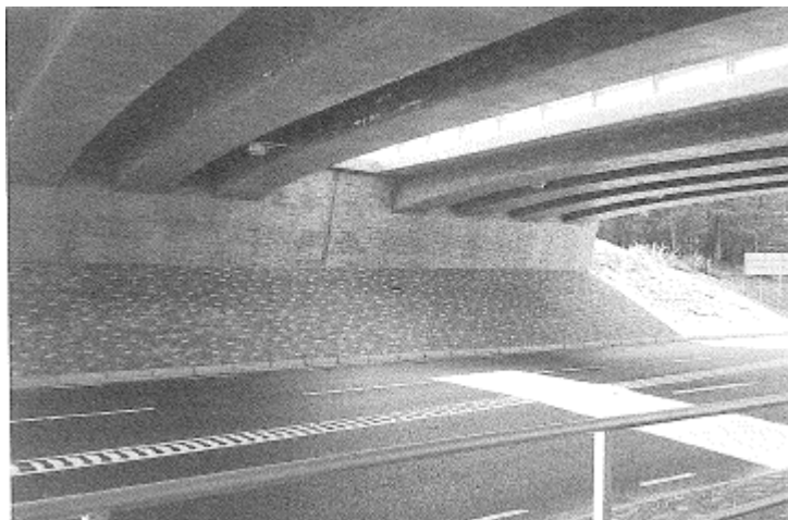
Figure 4.5 The beams are fixed into the abutments, from Vägverket (1996)
