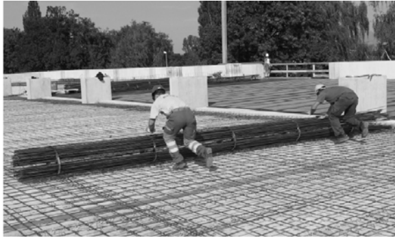
Figure 2.12 Prefabricated 'rolled' reinforcement (Bamtec 2011)
