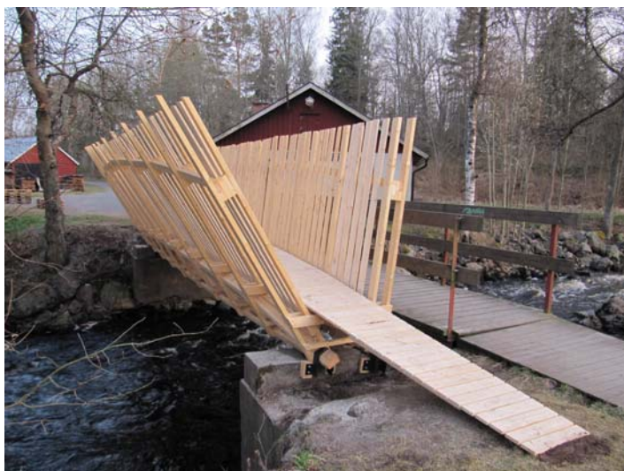
Figure 2.20 The completed bridge
