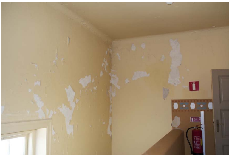
Photo 8. The paint is flaking off in one of the staircases on the north side of Teatern.
