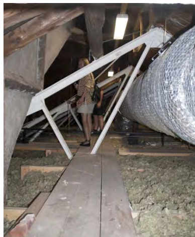
Photo 20. Teaterns vaulted ceiling as seen at the attic showing the wooden construction and steel construction and the added insulation. Photo Maja Lindman.
