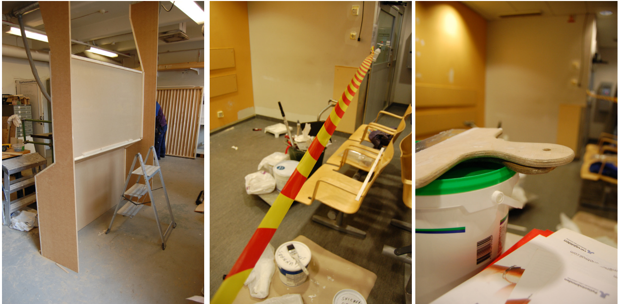
Figure 8.1 During the building and installation of the information module.
