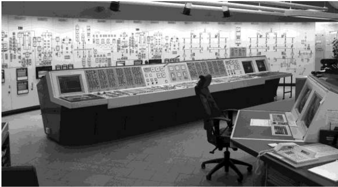
Figure 15 The turbine control desk at Ringhals 4
