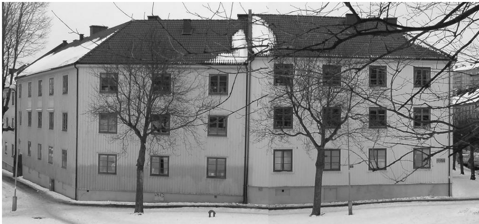
FIG 1. The studied multi-family building with ground floor masonry walls and first and second floor walls with structural wood (not shown here). The façade to the right of the firewall is retrofitted with vacuum insulation panels and the left façade is kept as reference.
