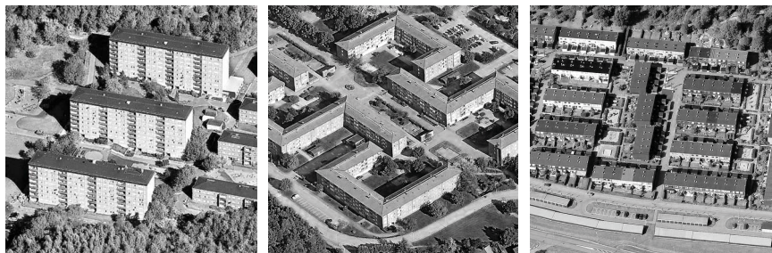
Figure 3. Three examples of building structures common in Million Homes Programme areas: (a) freestanding eight-storey slab blocks; (b) semi-enclosed yards with three-storey slab blocks; (c) two-storey row houses.
