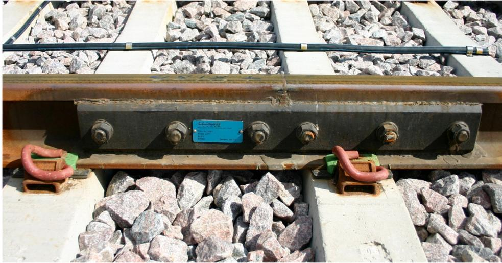
Figure 1.2: A photo of an assembled insulating joint.
