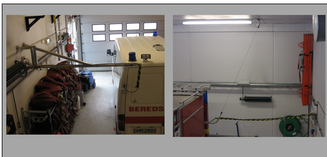
Figure 7-3 shows the two power construction on the fire trucks at Tjeldbergodden, which generate the possibility to drive away without manually unplug the power cable.
