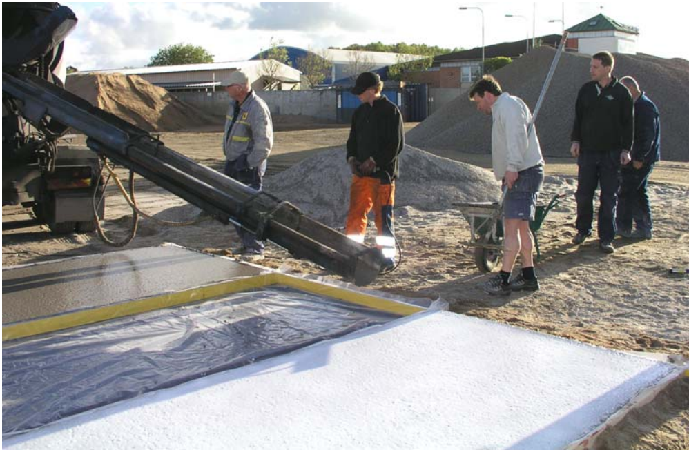
Figure 136. Casting of slab elements for the field study.
