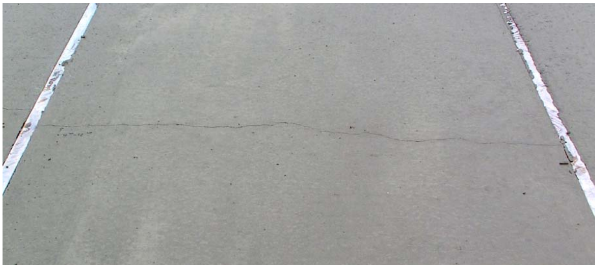
Figure 140. Picture showing a slab with a large crack.
