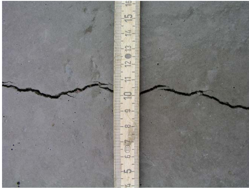
Figure 141. Picture showing a close-up a large crack.
