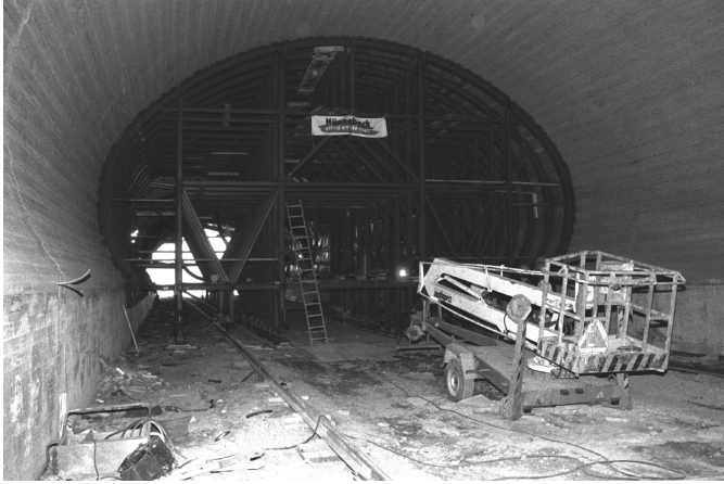
Figure 2. View of the tunnel lining cast with self compacting concrete.
