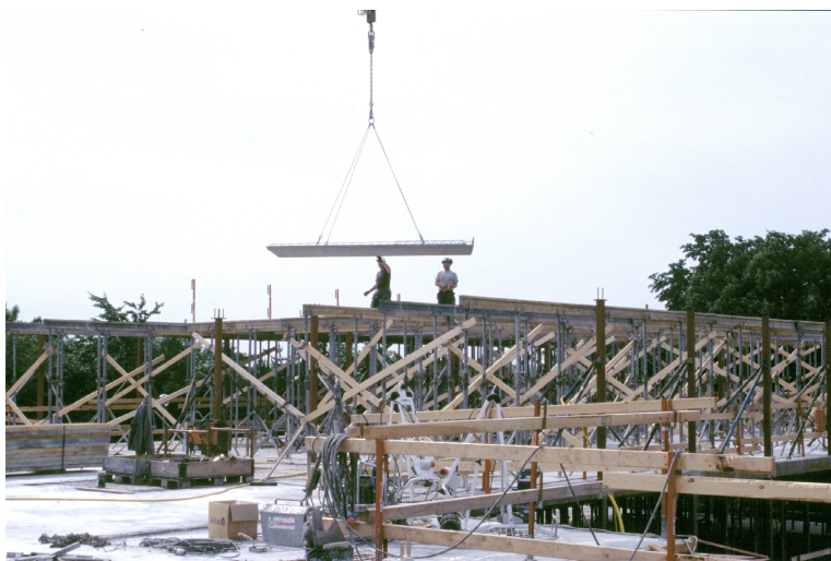
Figure 2. Erection of lattice girder element on the construction site.
