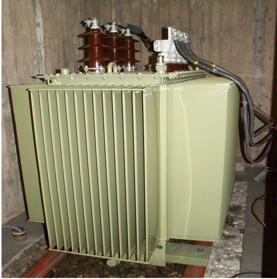
Fig.6.3 Windmill Transformer (TX1).
