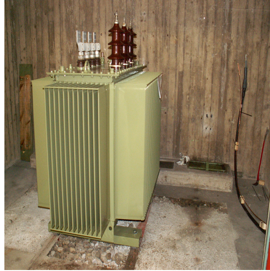
Fig.6.4 Load side Transformer (TX2).
