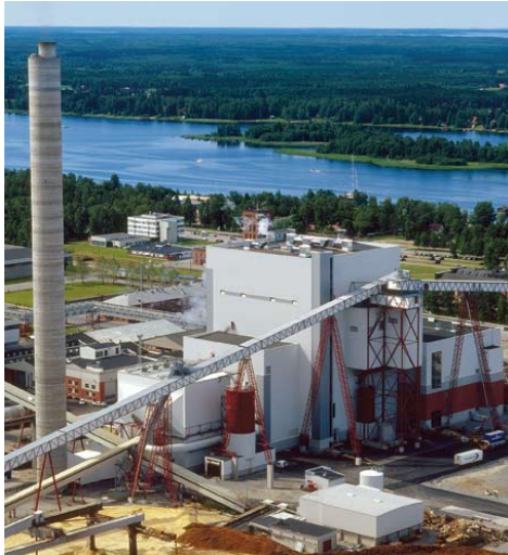
Figure 2: The world's largest (550 MW th ) biomass-fired CFB boiler in Alholmens Kraft (Finland). a. Photo of plant (courtesy of Alholmens Kraft, plant owner) b. Illustration of circulating loop (courtesy of Metso Power, manufacturer)
