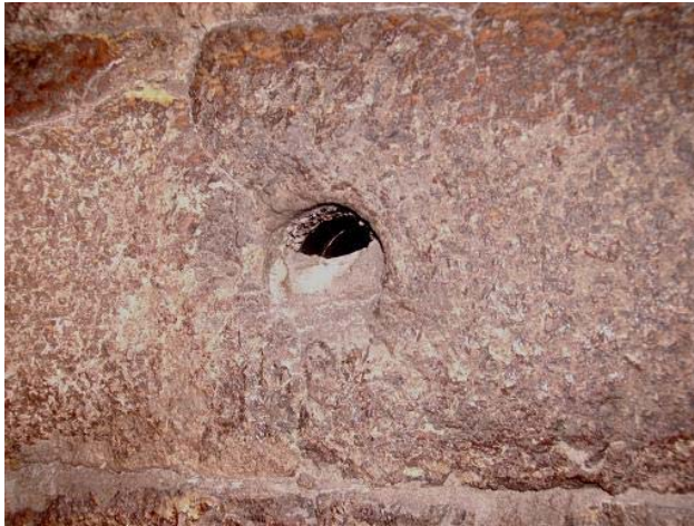
Figure 12: Partial blocking of a secondary air nozzle. Photo taken from inside the Chalmers CFB boiler.
