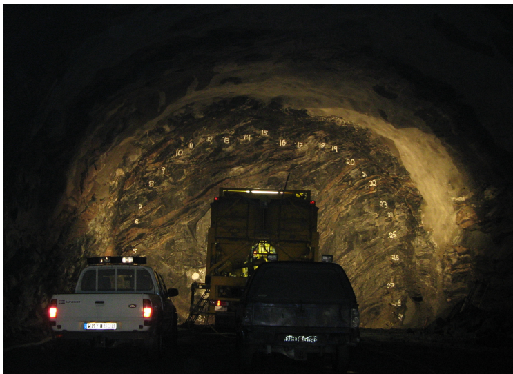
Figure 20. Grouting layout in field, Fan 1. The numbers represent the location of the grout-holes.
