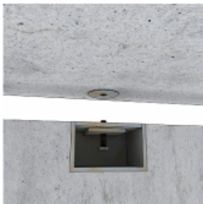
Figure 7.2 Intermediate floor element supported on wall element, Consolis (2007).
