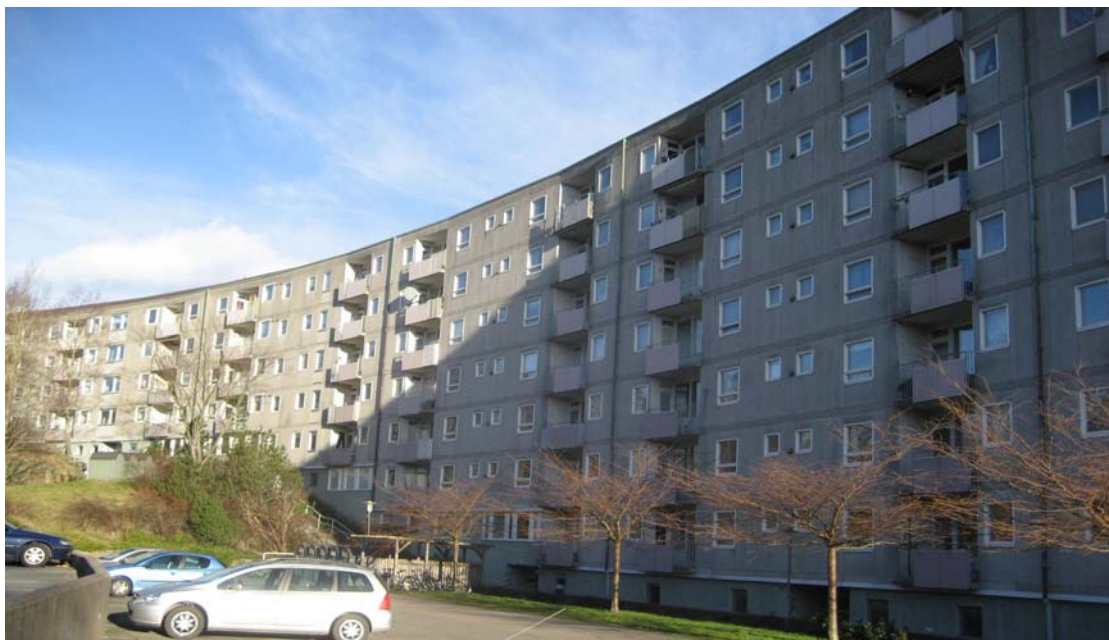
Figure 1.1 Typical house with prefabricated elements and visible joints from the post-war era.
