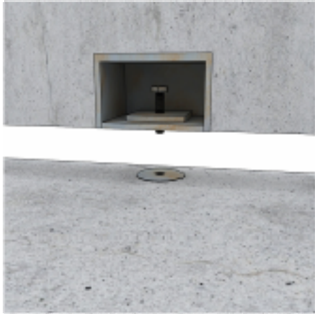
Figure 7.3 Wall element supported on floor element, Consolis (2007).
