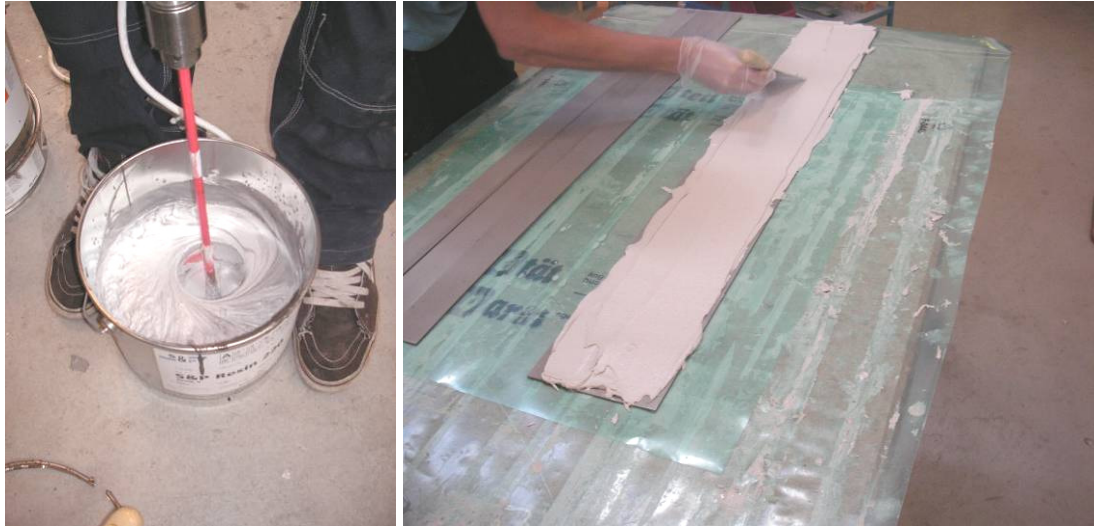
Figure 3.4 Mixing the epoxy (left), applying the adhesive to the laminates (right).
