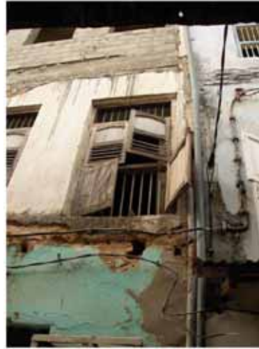
Figure 122 “Reparation” made with concrete instead of lime, which will cause blisters and cracks inviting fungi and insects to inhabit the structure.
