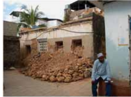
Figure 116 When the floor- and ceiling-bearing mangrove poles rot, the walls lose their foothold and tear apart.
