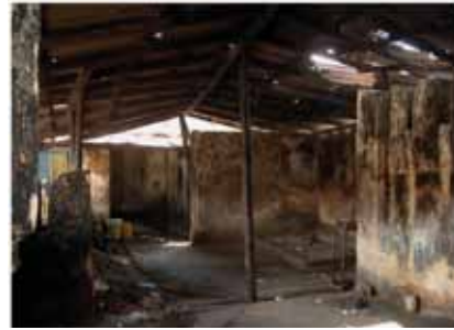
Figure 98 A kitchen installed on the rooftop covered with corrugated iron sheets prevents the intended cross ventilation of the evening sea breeze penetrating down the open courtyard into the inner rooms.
