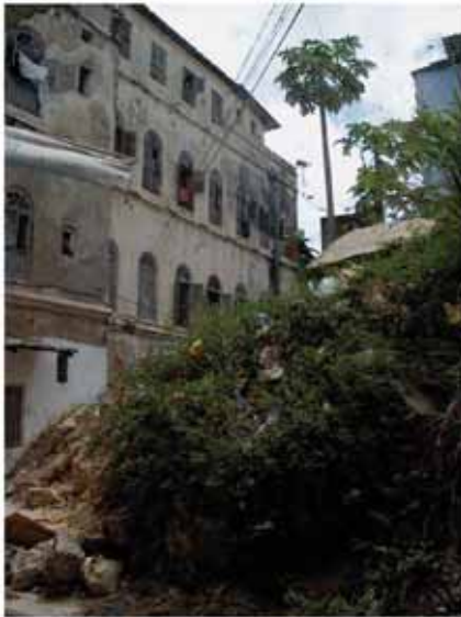
Figure 123 The picture shows Hurumzi house no. 234 a deteriorating behind a heap of stones and garbage, 1992.
