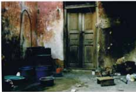
Figure 97 This photo documents the unhappy influence on the building structure of bringing the habit of making fire and food down on the ground up the second floor.
