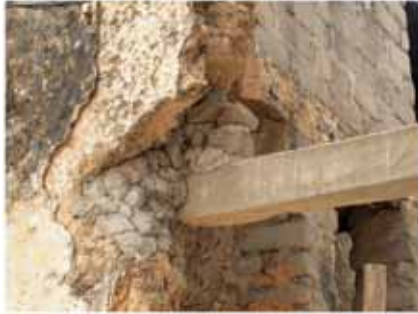
Figure 115 Repair mixing coral stones, lime, concrete and cement, the worst mixture of materials in a building structure founded on coral and lime.
