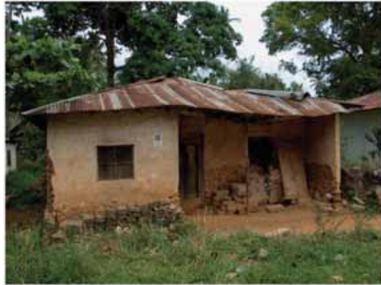
Figure 34 A Swahili house either under construction or near collapse.
