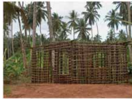
Figure 36 Swahili building construction.
