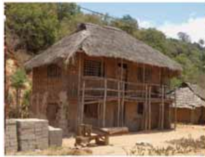
Figure 39 Outside Pangani on the North East coast of Tanzania this two-storey wattle and daub house was registered.
