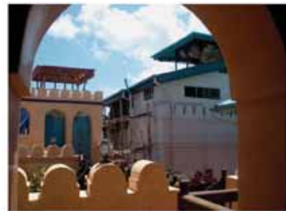
Figure 155 The photo taken in 2004 shows major ongoing repairs.
