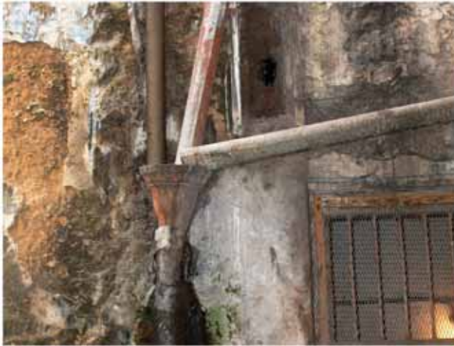
Figure 114 A typical attempt at repairing a leakage.
