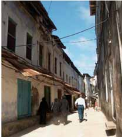
Figure 52 Indian shop-front row houses in Kajifjeni area in Zanzibar.
