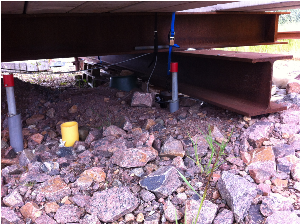
Figure 5.2: The loading rig beam on top of the thermal test pile after static loading test to failure. After failure, the pile head is displaced about 0.5 m downwards, ending at ground surface. Compare Figure 4.5 (before failure).
