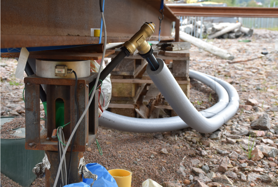
Figure 4.5: Pile head designed to let collectors, cables and fibre sensors pass in and out of the pile. Inside the piles a U-tube heat exchanger, made of high density polyethylene (HDPE) pipe, with 25 mm outer diameter was installed for exchanging heat with the ground. A load cell to measure data on applied static load is placed between the loading rig beams and the pile head.
