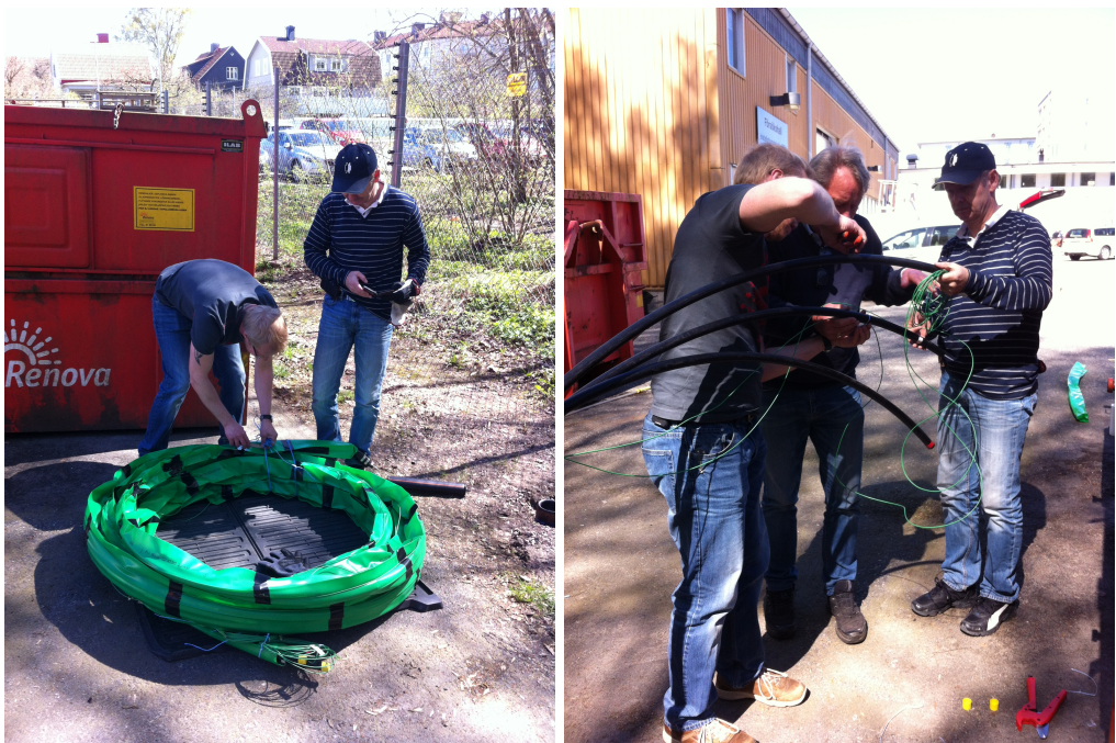
Figure 3.11: Preparation works at the test site at Chalmers Johanneberg Campus area. The exchanger pipes and fiber sensors are prepared, fixed together and rolled up before installation in the field.
