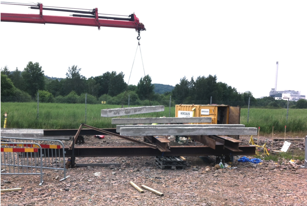
Figure 4.3: Loading rig under construction and loading. At the left part of the rig the foundation piles are endbearing, at the right side the piles are floating and are used in the thermal tests. The container behind is for housing computer, logger etc. The concrete test pile is installed out of the figure, to the left.
