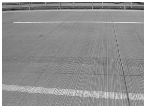
Figure 11. Newly (year 2004) laid cement concrete motorway pavement with unacceptable texture and thus unacceptable tyre road noise level (photos:Volker Schäfer, Brake).
