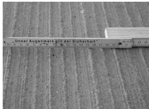
Figure 11. Newly (year 2004) laid cement concrete motorway pavement with unacceptable texture and thus unacceptable tyre road noise level (photos:Volker Schäfer, Brake).
