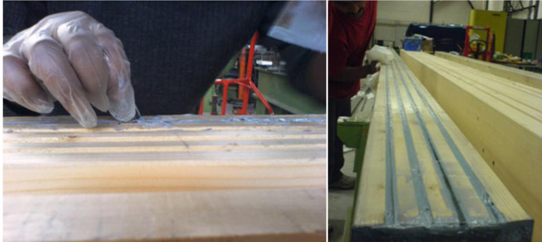
*Figure 5.7 Placing additional spacers to ensure straightness and even adhesive cover*
